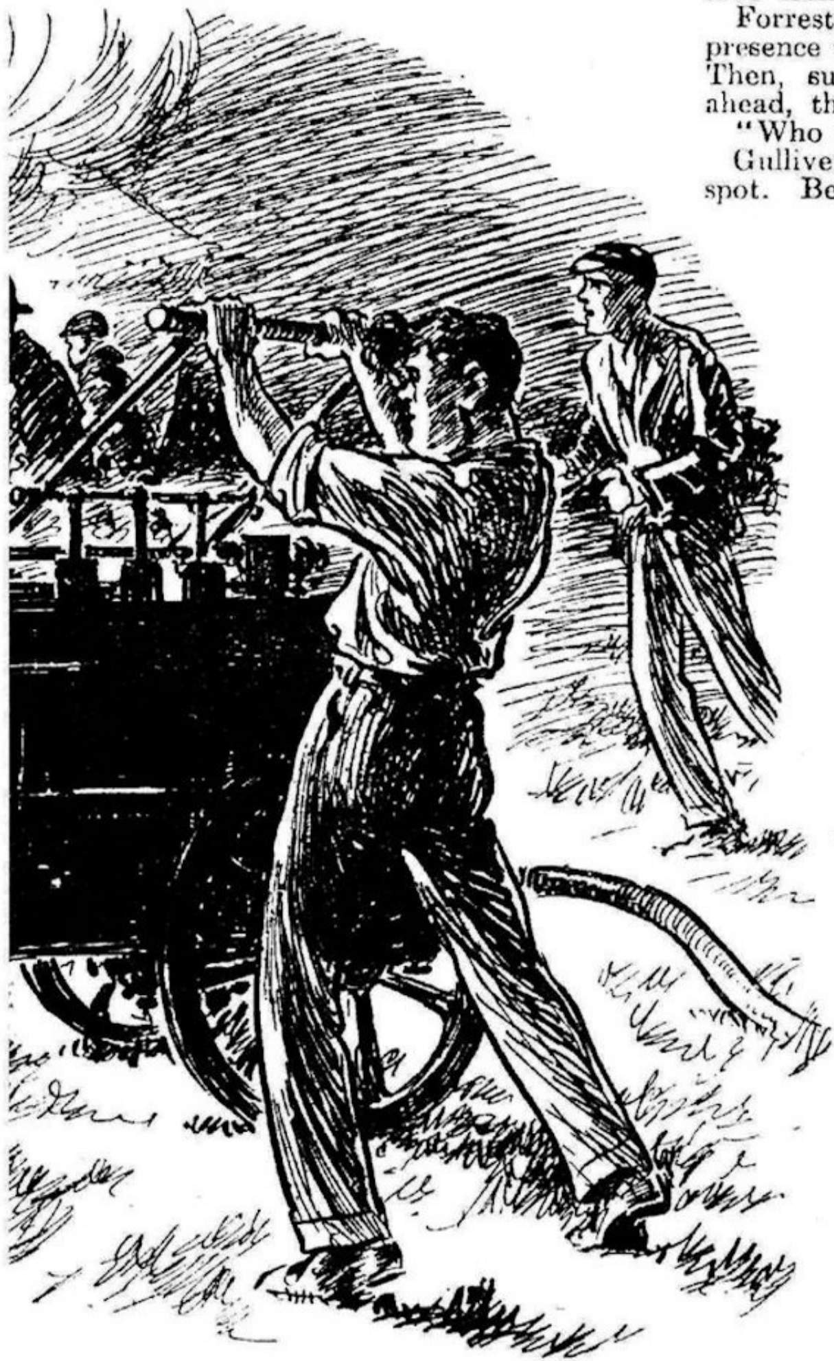
Pumping water from a brook, and with the hose played on vigorously to stop the flames from spreading to other stacks.
